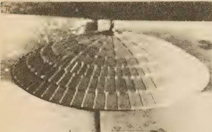
Hand Fabricating Large Plane Segmented Solar Energy Concentrating Mirrors
